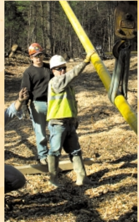
Pipeline crew at work
