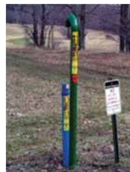
Pipeline markers are required by federal law and it is a crime to tamper with them.
