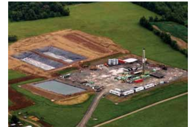
Shown are fresh water pits now used for water storage at drilling sites. The water pits greatly reduce truck traffic, reduce pollution and CO2 emissions and minimize disturbance to the public.
