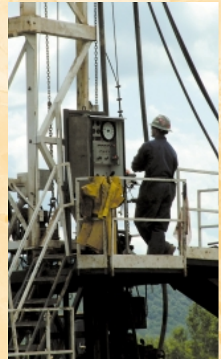
Crew monitoring completions rig
