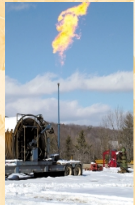
Flow and pressure testing
