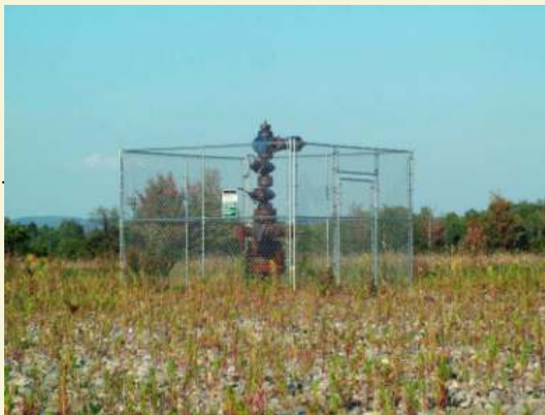
TEMPORARY SUSPENSION OF GANUNG #2 WELL IN TOWN OF DIX
